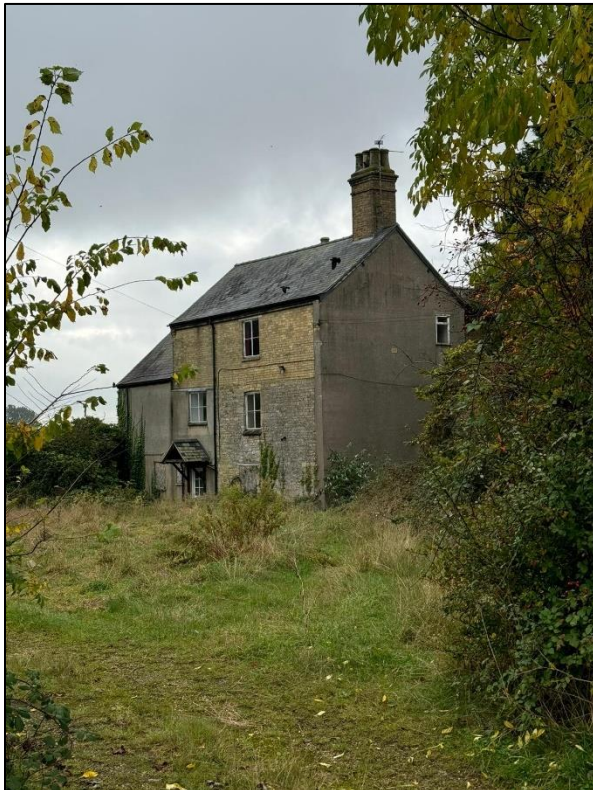
Plate 16: Temple Farm, Temple Road, which is built using the ruins of the tower that formed part of the Knights preceptory.
