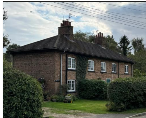
Plate 6: Brooklands, Middle Cottage and Harrison. It is pleasing to see that a good number of the Yorkshire sliding sash windows have been retained.
