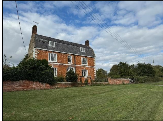
Plate 12: Moorfield House Farm, located on a slight rise contributing towards its prominence. It is constructed of a mix of brick and limestone with a later brick extension to the rear.
